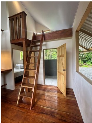
The custom ironwood ladder to the loft — one of several pieces built for this house.
