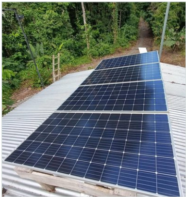
The 1,480 W array on the ridge, angled for the equatorial sun.
