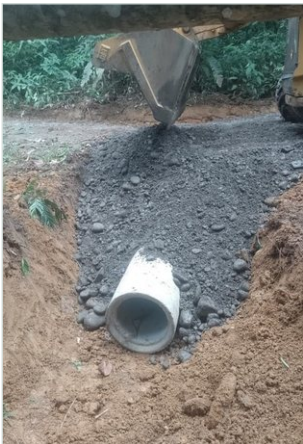
The easement road under construction — one of the seven 75 cm culverts going in. This is why the road carries traffic through the rainy season.
